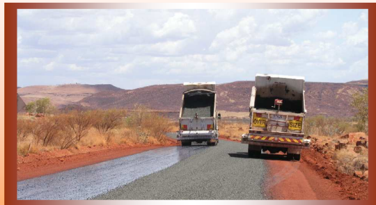
Resealing of Roebourne - Wittenoom Road
